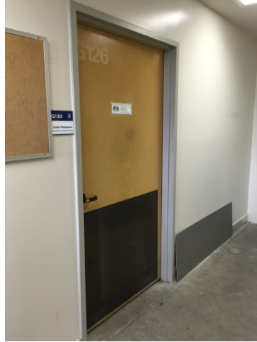
Interior Door, Rm 130
