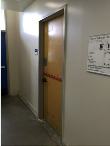
Interior Door, Rm 129
